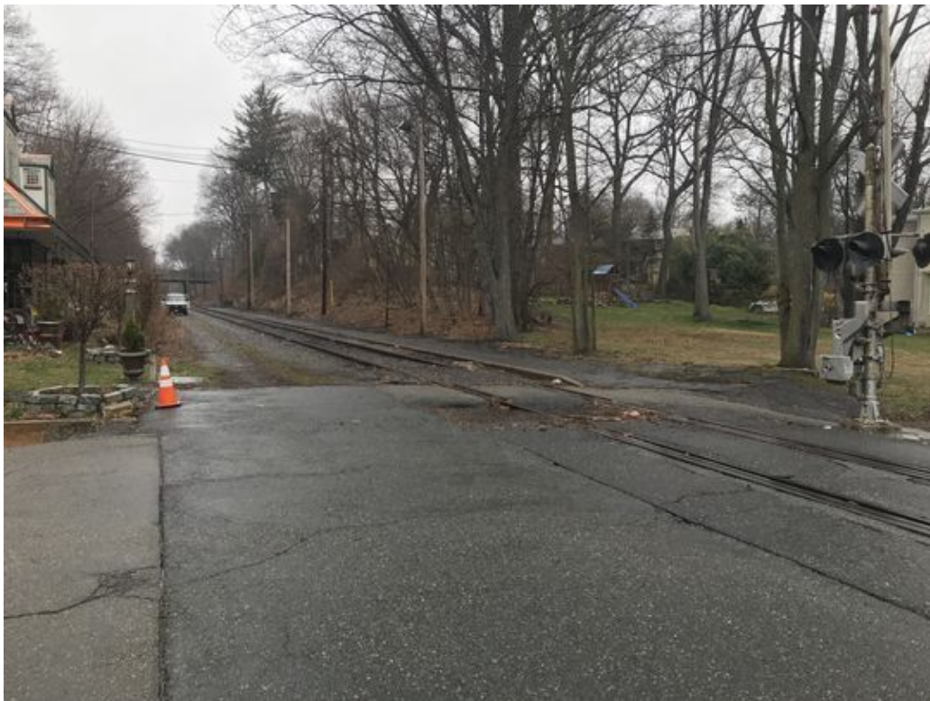
This section of the old Boonton railroad line, being envisioned for a greenway, is located in Glen Ridge. (Photo: Ricardo Kaulessar/NorthJersey.com)
