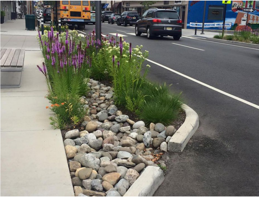
Stormwater Planter, Millburn, NJ
