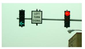
Use of concurrent, protected/permissive, or protected left turn phasing provide increasing levels of conflict reduction between vehicles and pedestrians using a parallel crossing.
