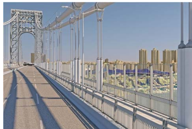
New 11' high safety fence at the main span of the bridge; sidewalk access ramps will be 9' high; vehicular side rail will also be replaced
