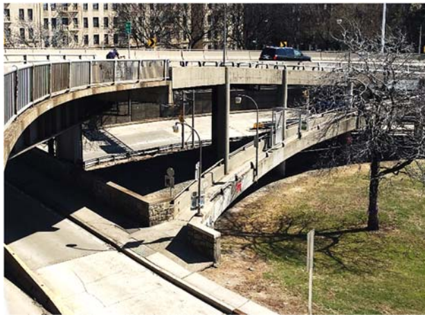
Existing condition at NY-South: W. 178 th Street and Cabrini Boulevard: absence of entry area and street buffer; ramp access to bridge is narrow with constricted turns
