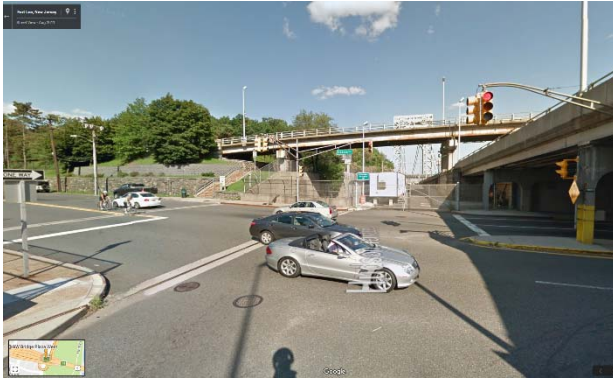
Existing condition at NJ-North: Hudson Terrace looking east: absence of crosswalk, entry area and street buffer; stair-only access to bridge
