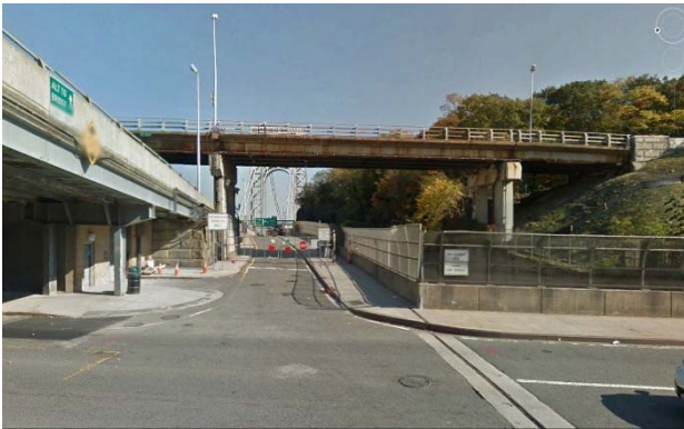
Existing condition at NJ-South: Hudson Terrace looking east: absence of crosswalk, entry area and street buffer; narrow sidewalk with vehicular gate impediment
