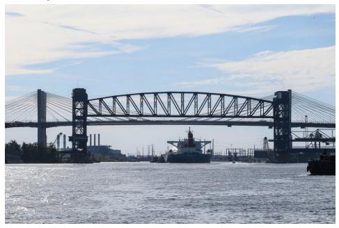
A view of the Arthur Kill Vertical Lift Bridge from the north, with the Goethals Bridge behind it. The Arthur Kill bridge, built in 1959 for rail cargo, is the longest lift bridge in the world, according to Encyclopedia Britannica, with a truss span 558 feet long.
